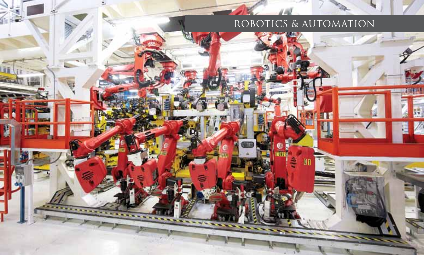
FCA Melfi plant (Italy). 18 Robot Open RoboGate.
